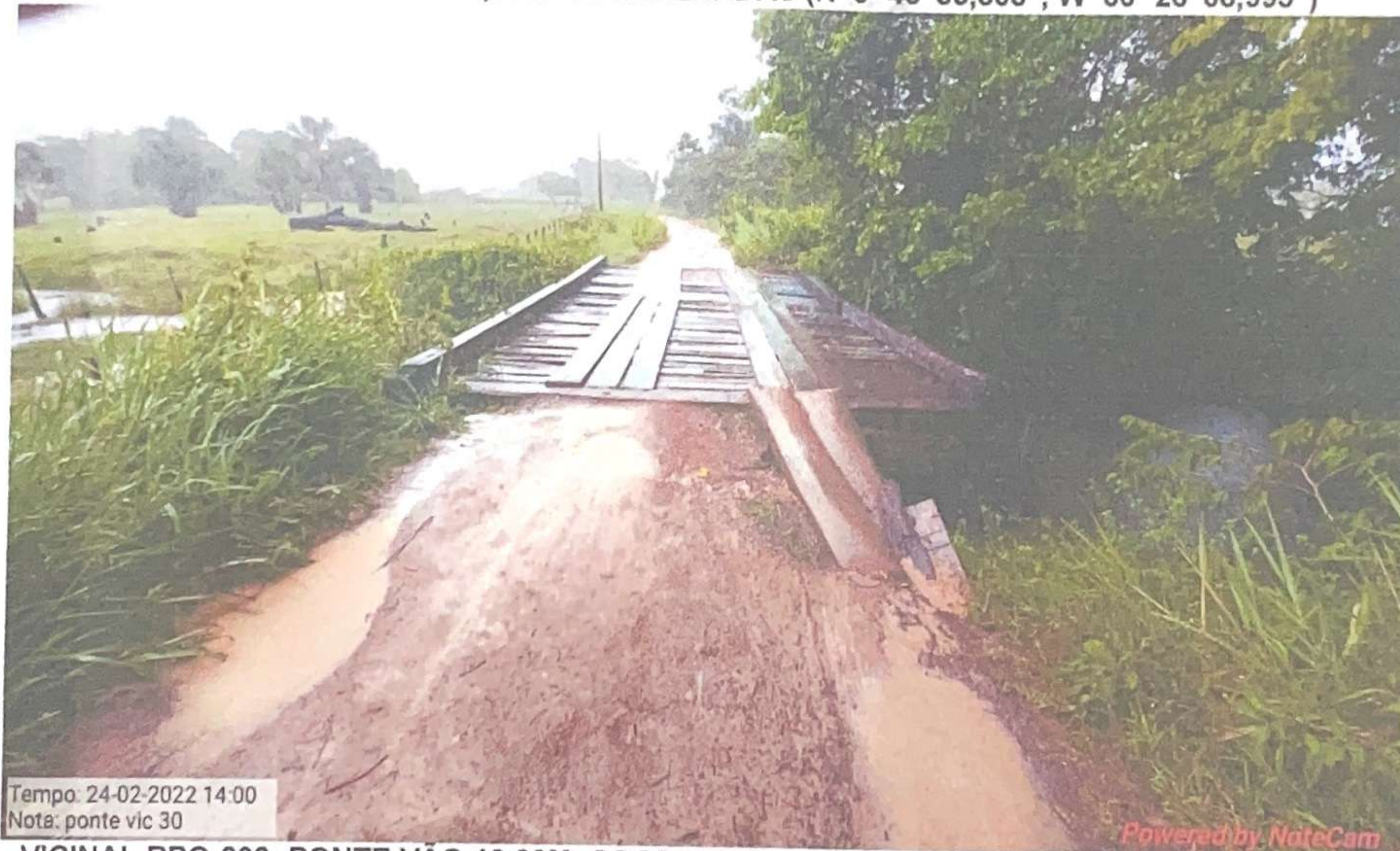
VICINAL RPO-262: PONTE VÃO 10,00M COORDENADAS (N 0° 43' 25,676"; W 60° 23' 34,694")
